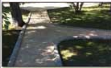
ROUND MOLD NO COLOR OR TEXTURE ADDED - 1/4 DOWN LIMESTONE FILL
